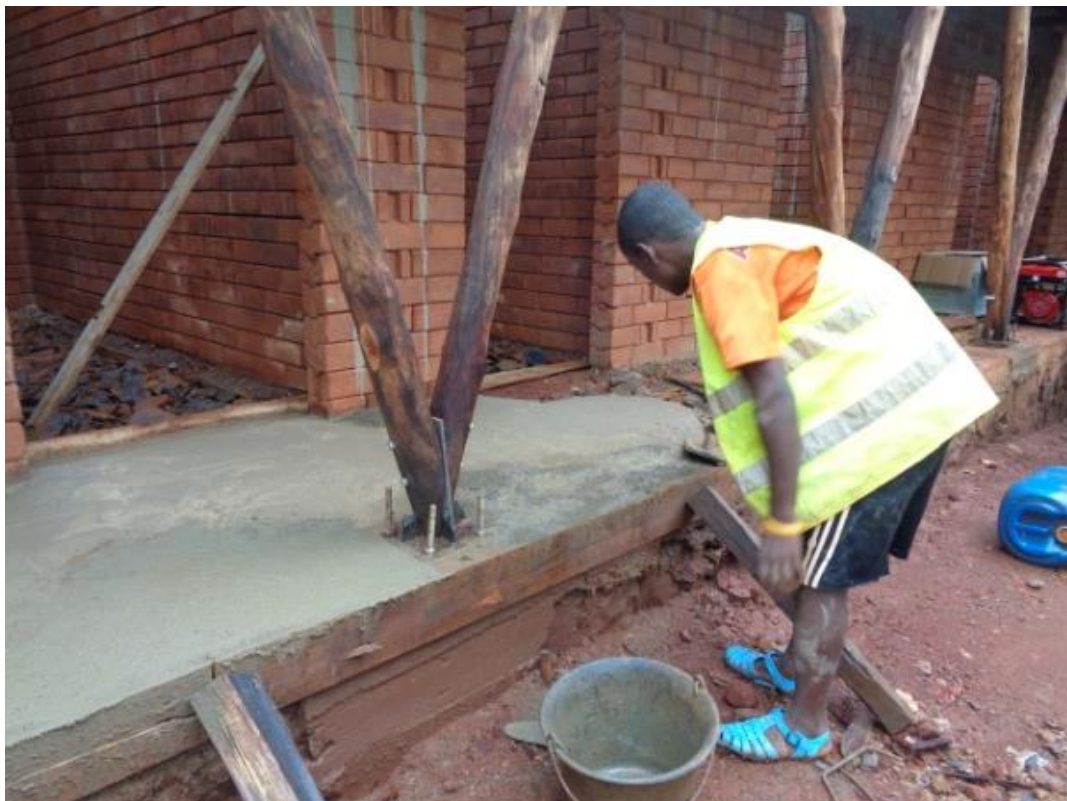
Photo 17 : Concreting the floor
