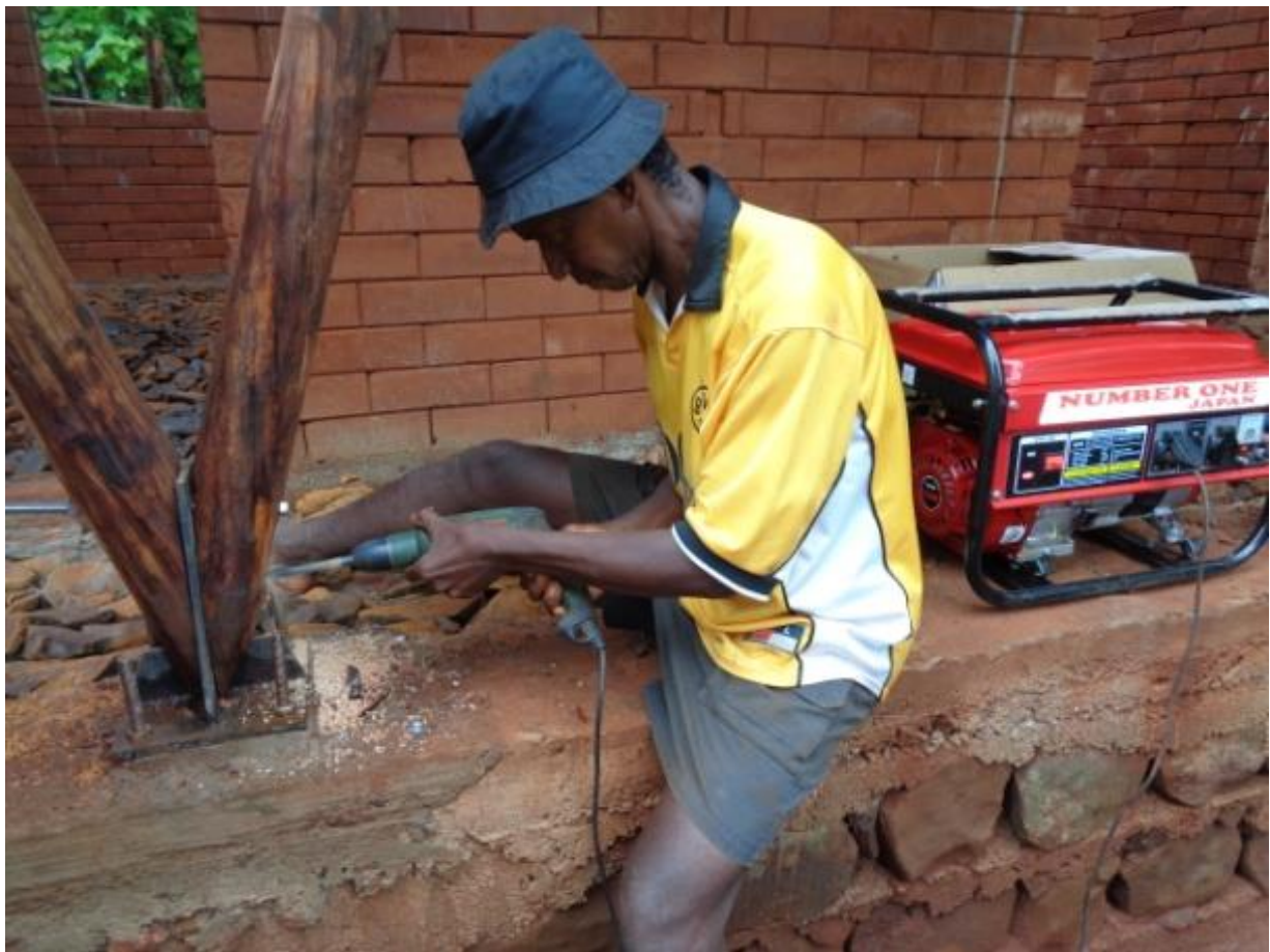
Photo 18 : Securing poles with threaded rod
